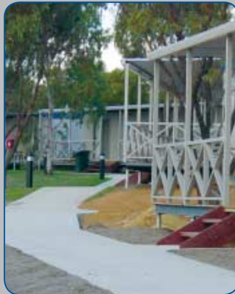
Accommodation Facility Ravensthorpe Joint Venture
